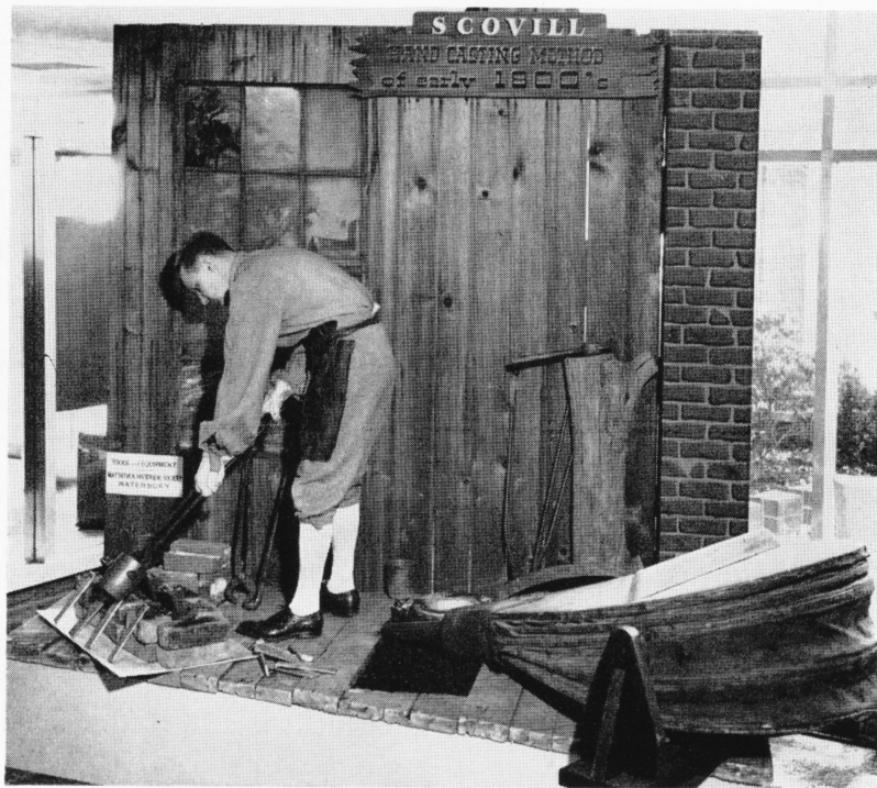
tion—and main theme of the 61 Connecticut Industry exhibits—was the re-enactment of America's first practical brass casting method (right). George Sunderland is shown pouring metal into a tiny 1-lb capacity mold.
